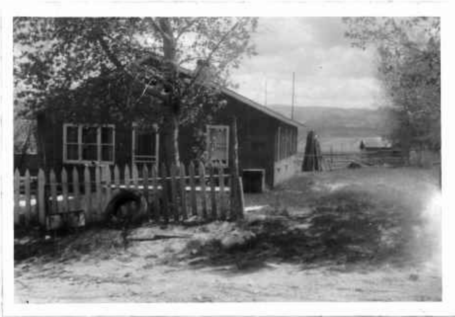
Fig. 29.-The site of the first Manila School
